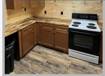
Maloney kitchenette renovated
