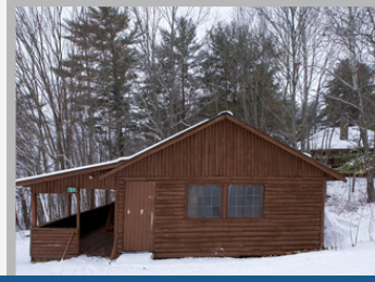
Rangers 1 lifted and leveled
