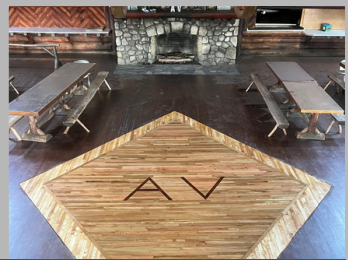
Dining Hall Floor Repaired
